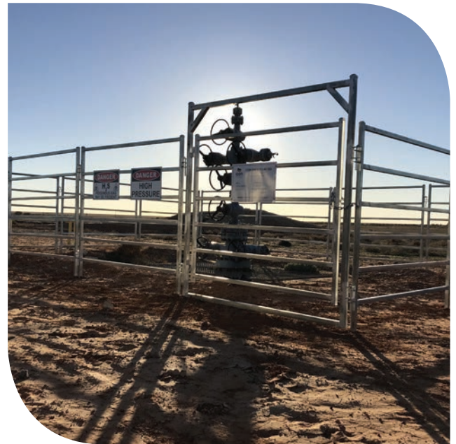
Image: Fencing around Halifax-1 wellhead
